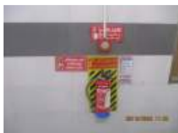
Fire Alarm Call Point & Fire Extinguisher.JPG
